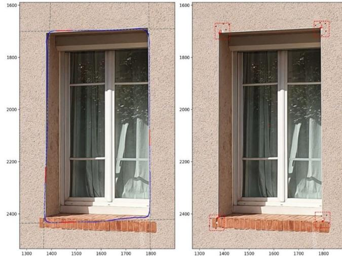
**Figure 4.** Illustration of the detection mask clean-up process with on the left in blue the original mask, in red the four tangents that explain most mask vertices, their extension in gray. On the right the intersection of these extensions is displayed in white with a search area around them in which several Harris corners are identified, in bright red the closest to the search area center is indicated, which is selected and indeed corresponds to the corner of the actual window void.
