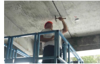
Figure 5 Hammer sounding inspection
