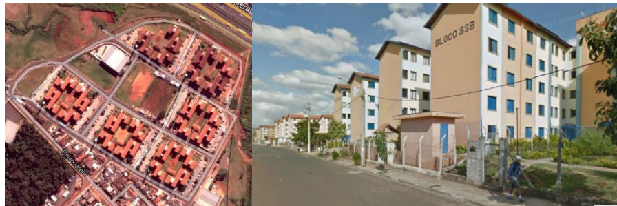
Figure 3: Aerial and street view of the social housing Campinas F – CDHU
