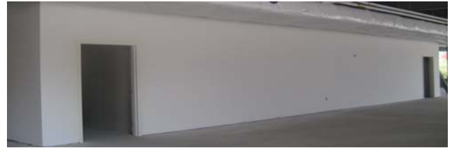
a) Picture of a concrete wall (14')
