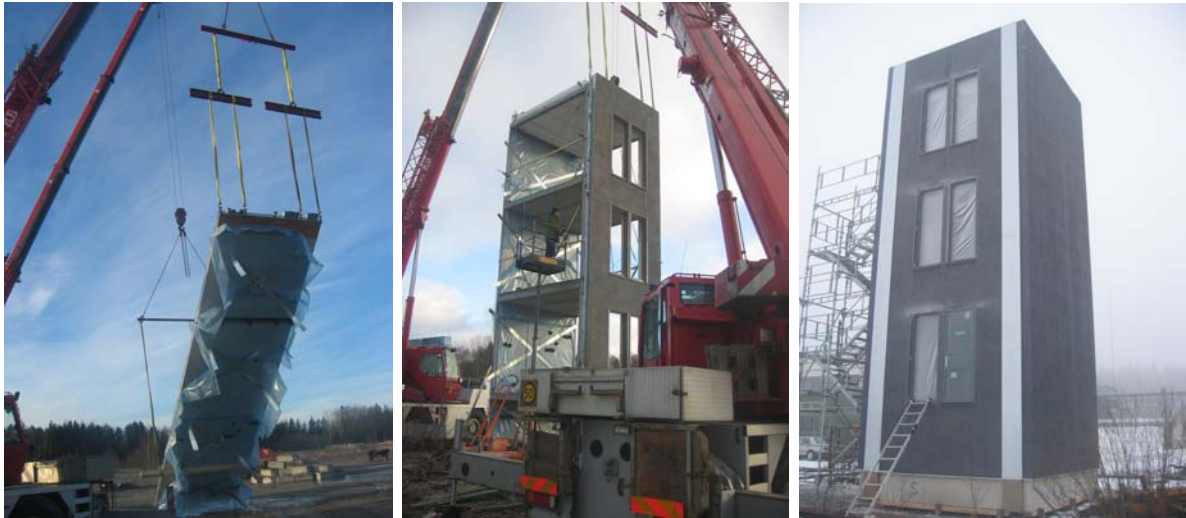
Figure2. assembly of the outer wall elements, the revealed joint elements can be seen in the picture to the right.
