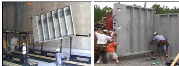
Figure 1: Precast Panel Wall System
