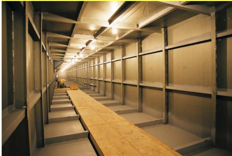
Figure 3: Lighted walkway within a Tay Road Bridge girder box
