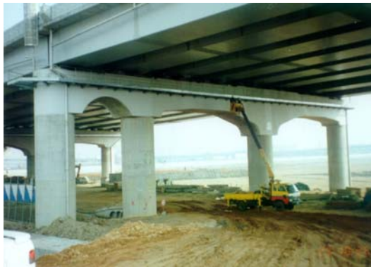
Figure 2: Inspection of bean lifter
