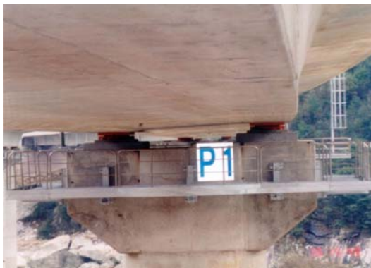
Figure 4: Built-in facility at coping
