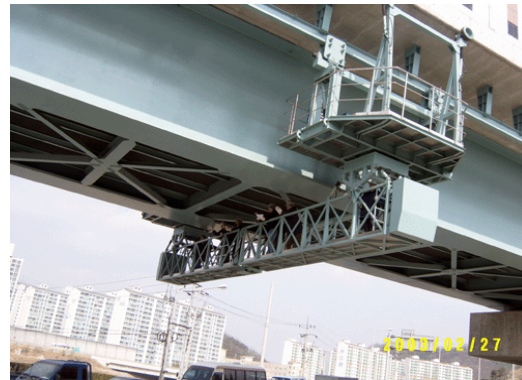
Figure 5: Movable system installed under deck
