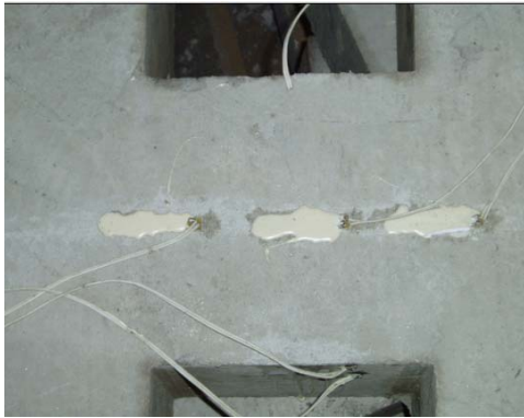
Fig.5 No Apparent Crack on the Load End of Concrete after Experiment
