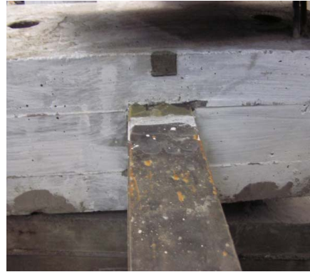
Fig.6 No apparent Crack on the Surface of Concrete of Bond Zone after experiment
