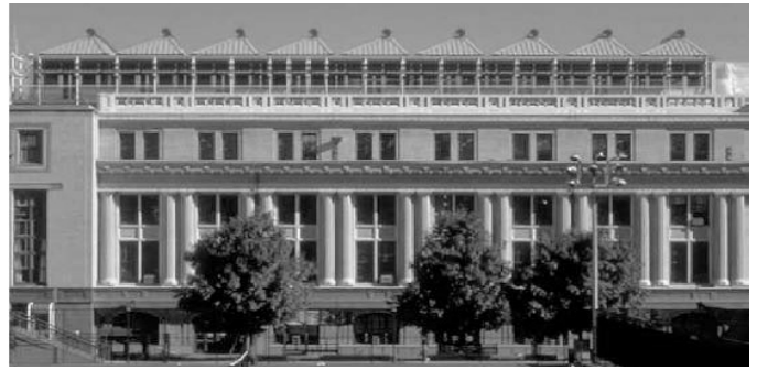
Figure 1. The Intelligent Workplace™, a rooftop extension of Margaret Morrison Hall at Carnegie Mellon University
