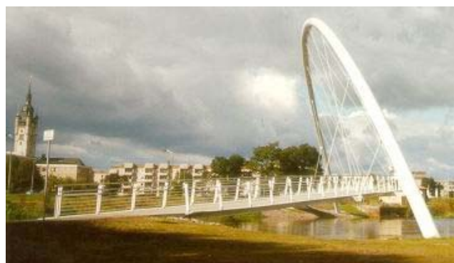
Figure 2 Arched bridge over the river Mulde in the city of Dessau (Germany)
