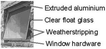
Figure 1: Components of an Aluminium Window
