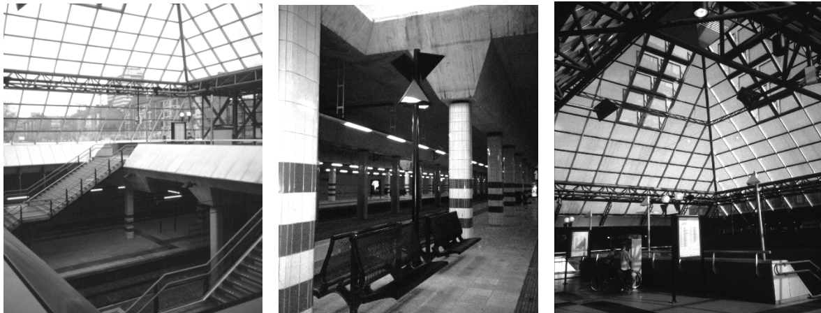
Figure 5, 6, 7: Rijswijk train station-atrium area (5), platform (6) and entrance level (7)
