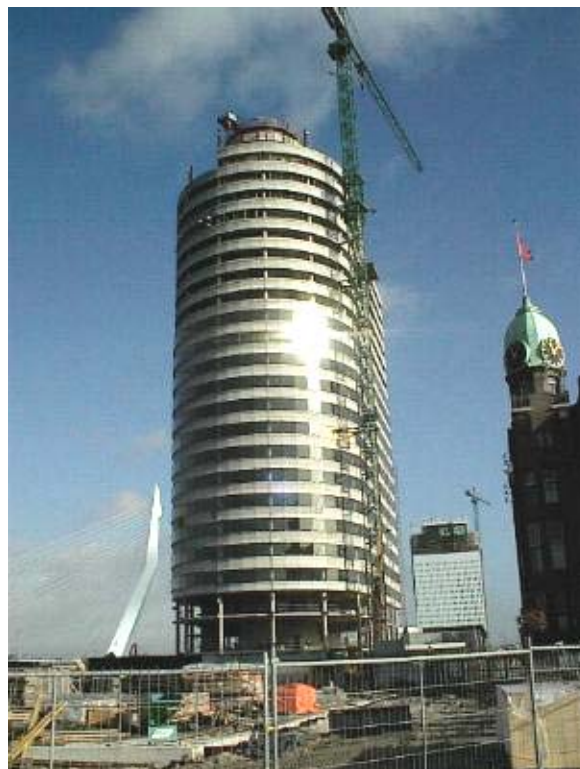
Figure 7. World Port Centre (under construction)
