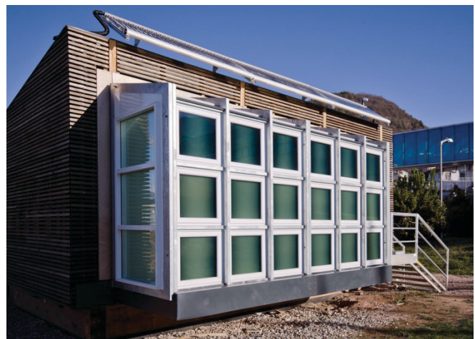
Figure 1: Exterior view of the openable south façade of the prototype house in Trento, N. Italy.
