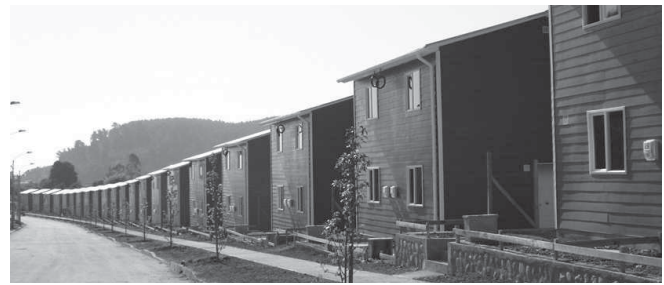
Figure 2: Highly repetitive housing typology as a result of a heavily prescribed design space (source: Author)
