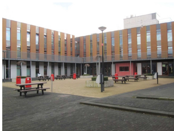
Figure 3 View on courtyard
