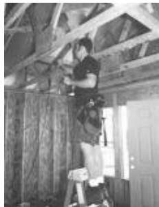
Figure 4: Builder Working on an Electrical System
