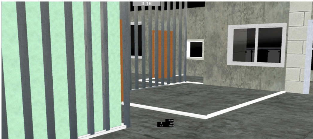
Fig. 2: Interior view of a virtual apartment, showing markings on the floor (at right), built studs (center) and studs with one side of boards built (at left).
