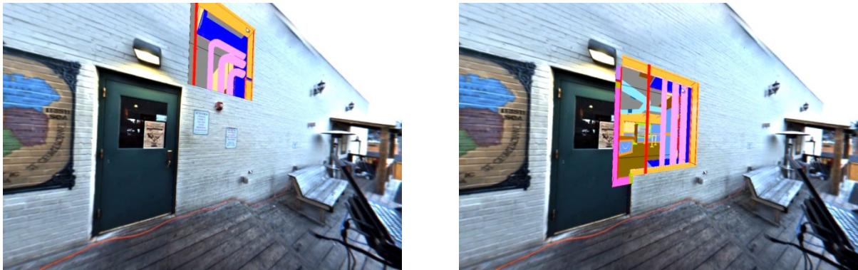
Fig. 9: Two frames extracted from the wall augmentation experiment. Virtual excavation reveals pipes hidden inside the wall and other elements inside the pub.
