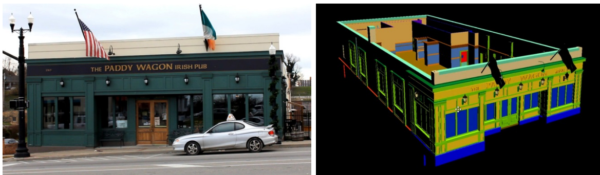
Fig. 4: The test site (left). The detailed 3D CAD model of the pub (right).
