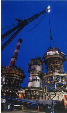
Fig. 2(a): Reactor lifting
