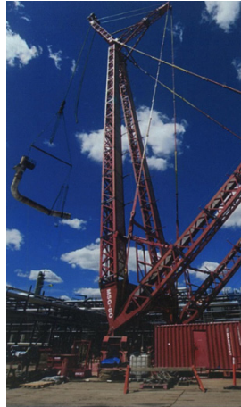
Fig. 2(b): Pipe 1 lifting
