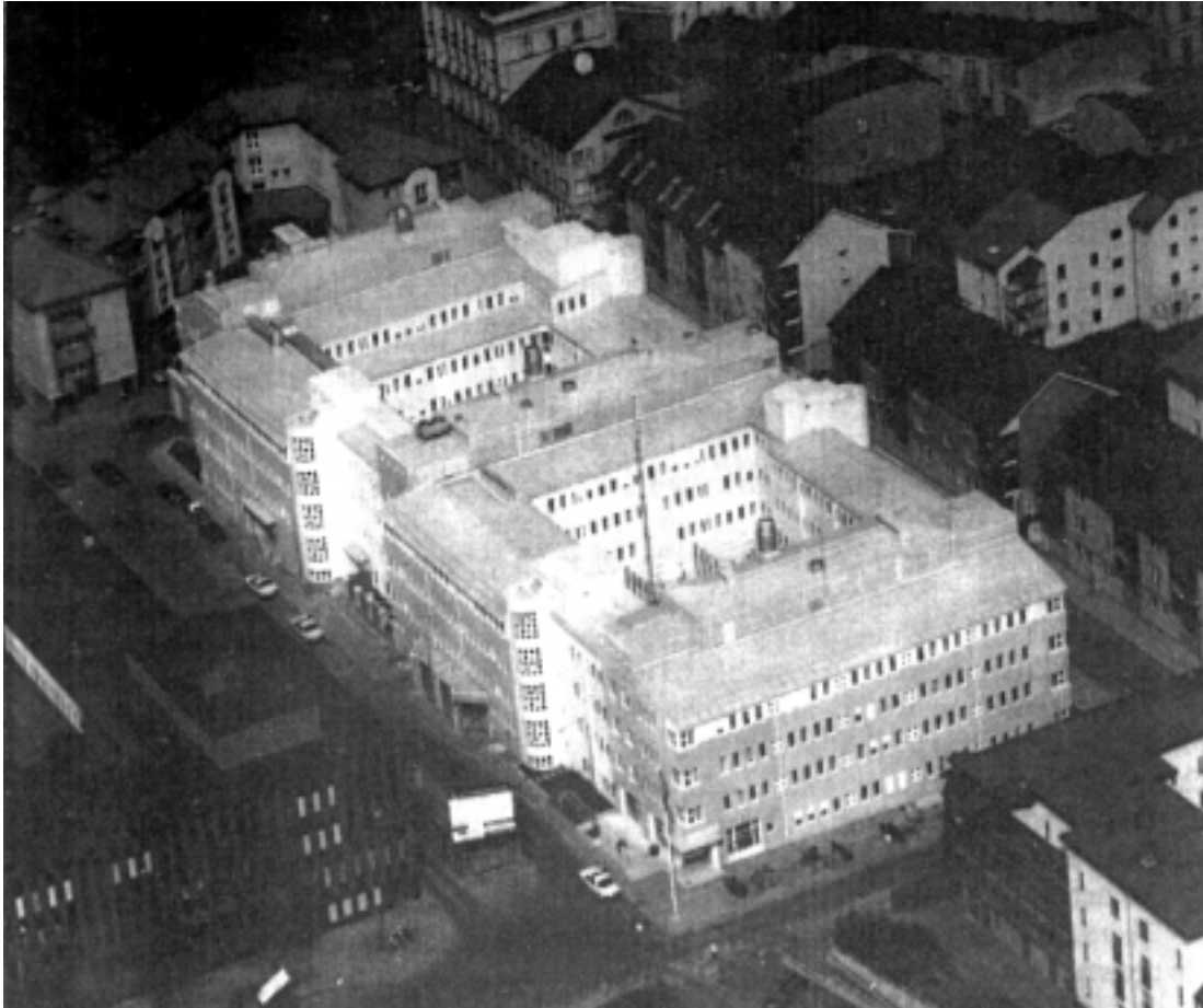
Figure 7:10 The test building of the Blandaren prototype
