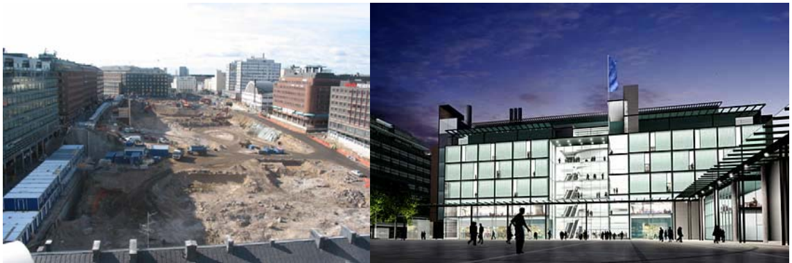
Figure 8 During and after construction
