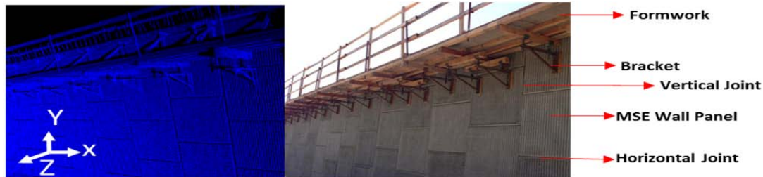
Figure 1. MSE Wall's Point Cloud and Image
